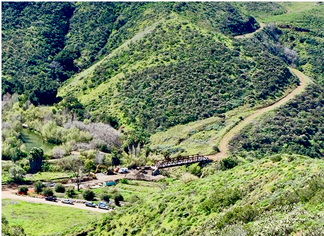
The Conejo Canyons Bridge seen from the Lizard Rock Trail.
